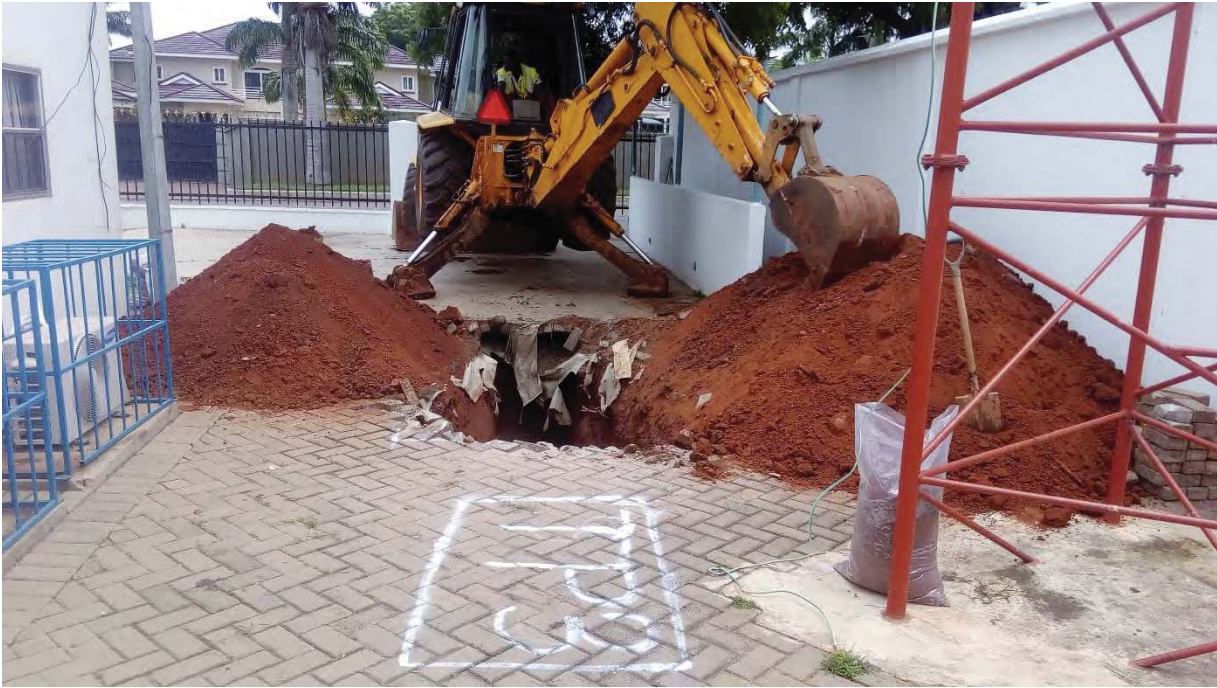
Plate 5 : Sinking of Trial Pit at TP3
