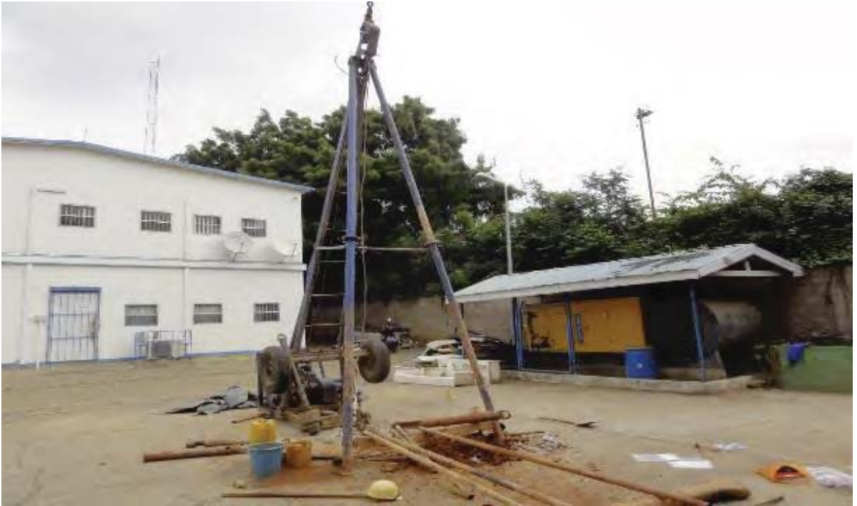
Plate 2 : Percussion drill rig positioning at location BH6
