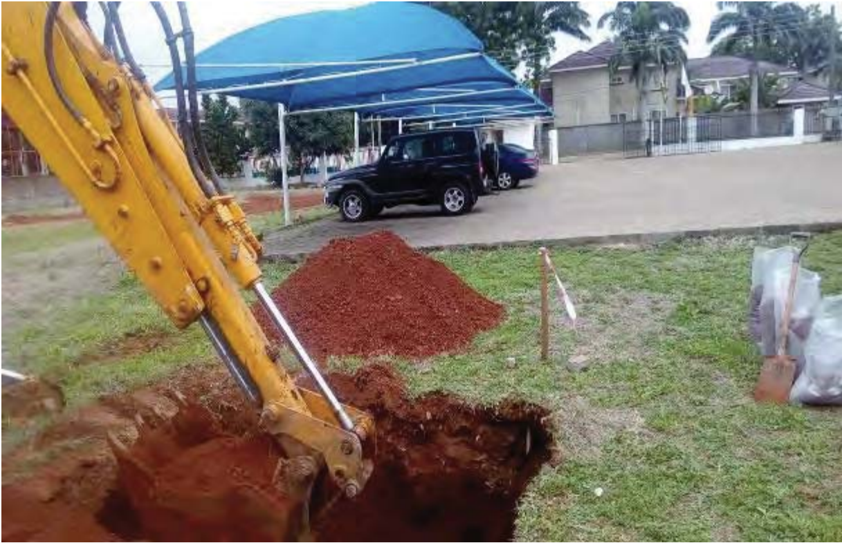
Plate 3 : Sinking of trial pit at TP1
